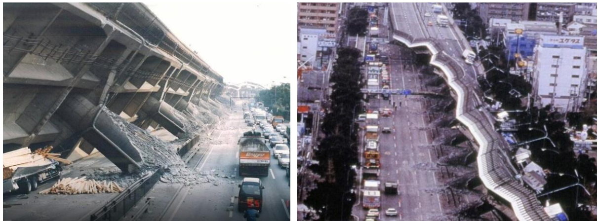
Figure 2. The collapse of the Fukae Viaduct on the Hanshin Highway [9, 10]
