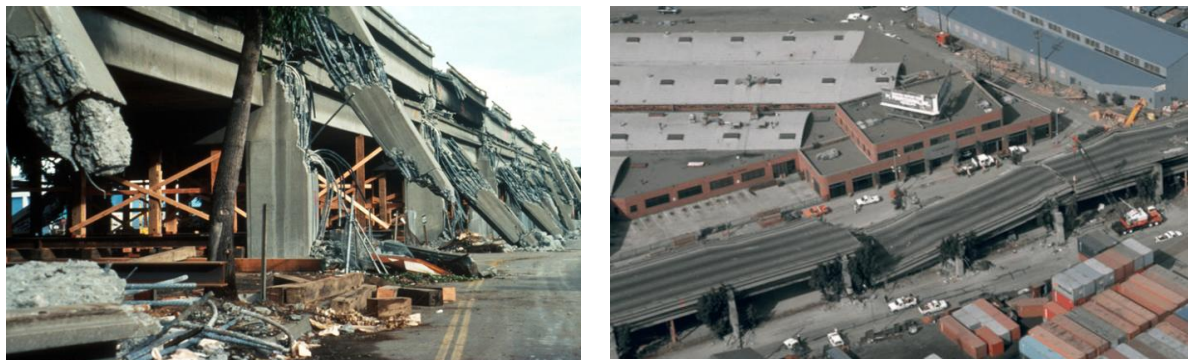
Figure 1. The collapse of the Cypress Street Viaduct during the Loma Prieta Earthquake [4, 5]
