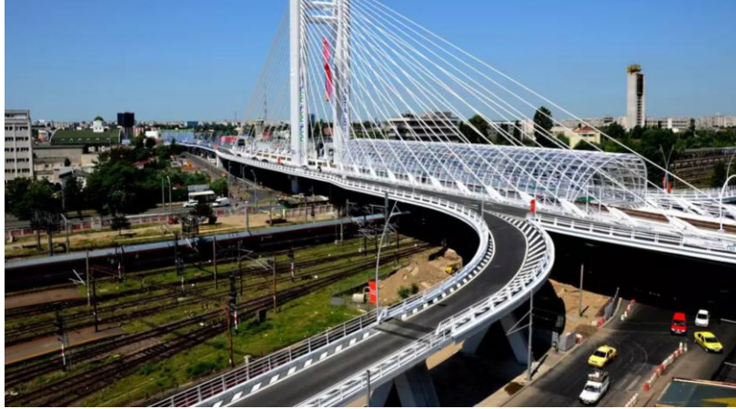
Figure 3. Basarab Overpass – the cable stayed bridge over the railway
