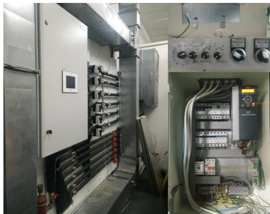
Fig. 30 – The hydraulic circuits of the climatic chamber
