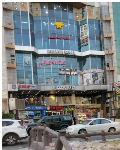
a. Picture of the building
