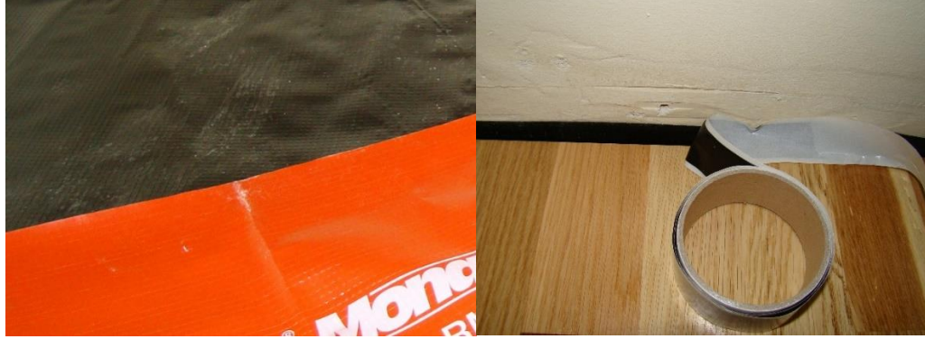
Figure 10 – Radon proof membrane and joint wall-floor sealing
