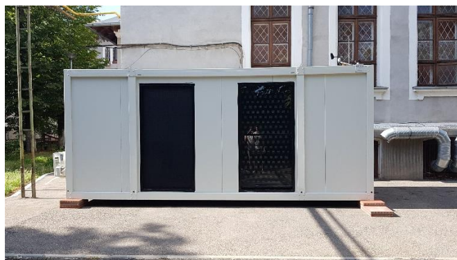
Figure 30. Container with integrated Solar Air Collectors
