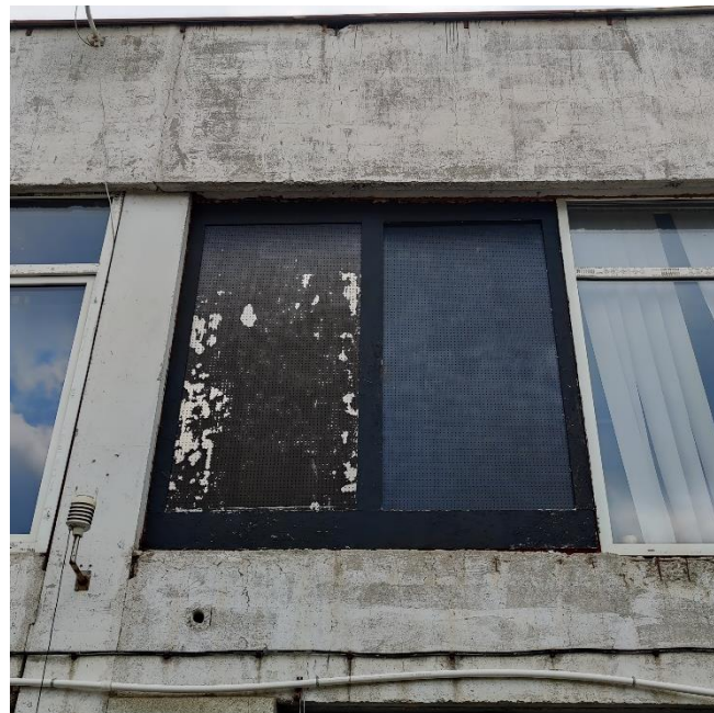
Figure 33. Solar façade after 2 years (left), new solar façade (right).
