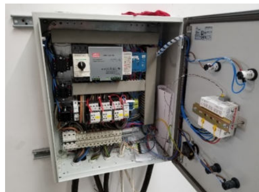
Fig. 10 (Figure 4.3): The electric cabinet for the bench and electric motor control.
