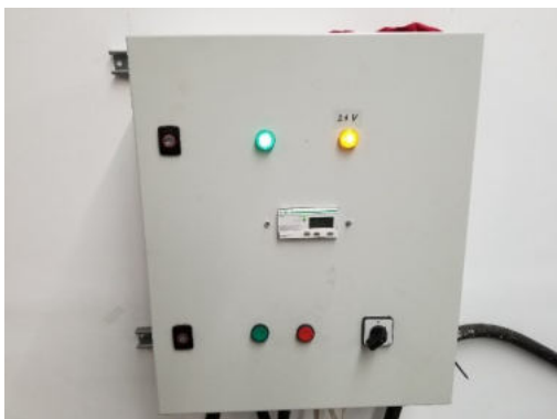
Fig. 10 (Figure 4.3): The electric cabinet for the bench and electric motor control.
