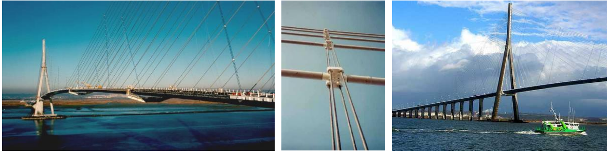
Figure II-2 – Cross ties on the Normandy bridge (Wikipedia, 2019)
