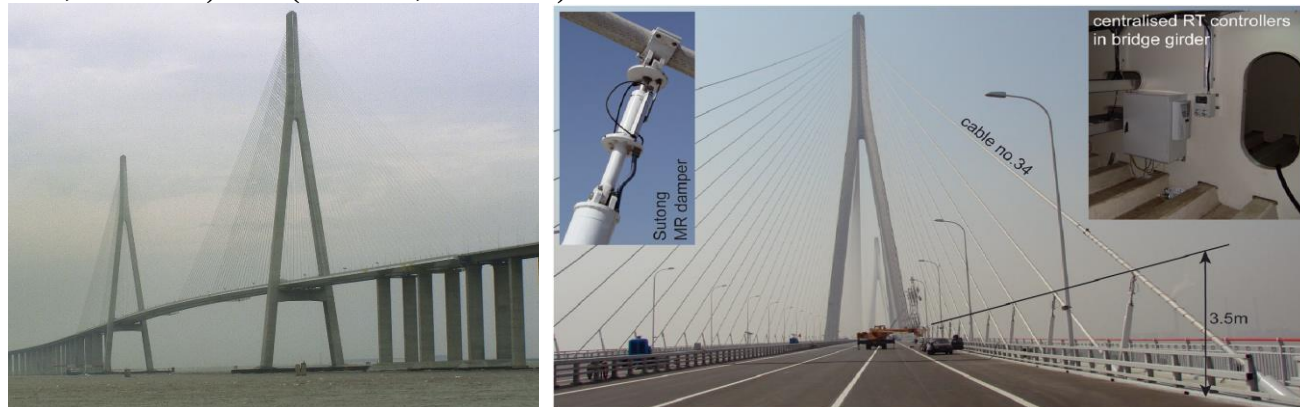
Figure II-13 – Dampers installed on the Sutong Bridge, China (Felix Weber H. D., 2014)
