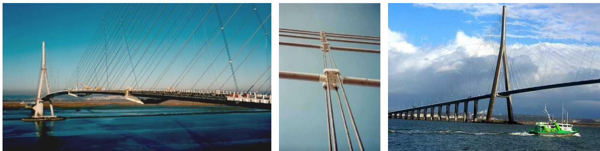
Figure 17 –Cross ties on the Normandy Bridge
