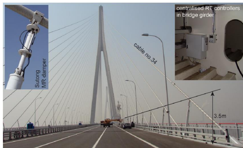
Figure 33 –Dampers on Sutong Bridge, China
