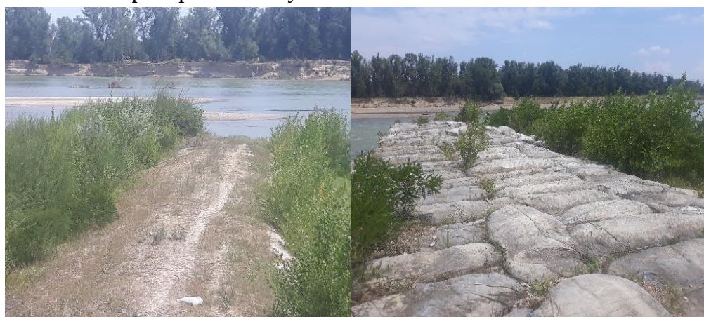
Fig.9.10. Development of spontaneous plants and shrubs in the areas with geocontainer works
