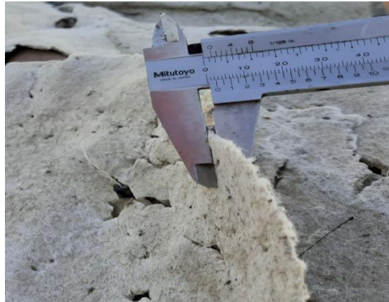
Fig.7.5. Geotextile degraded by U.V. and alluvium transport
