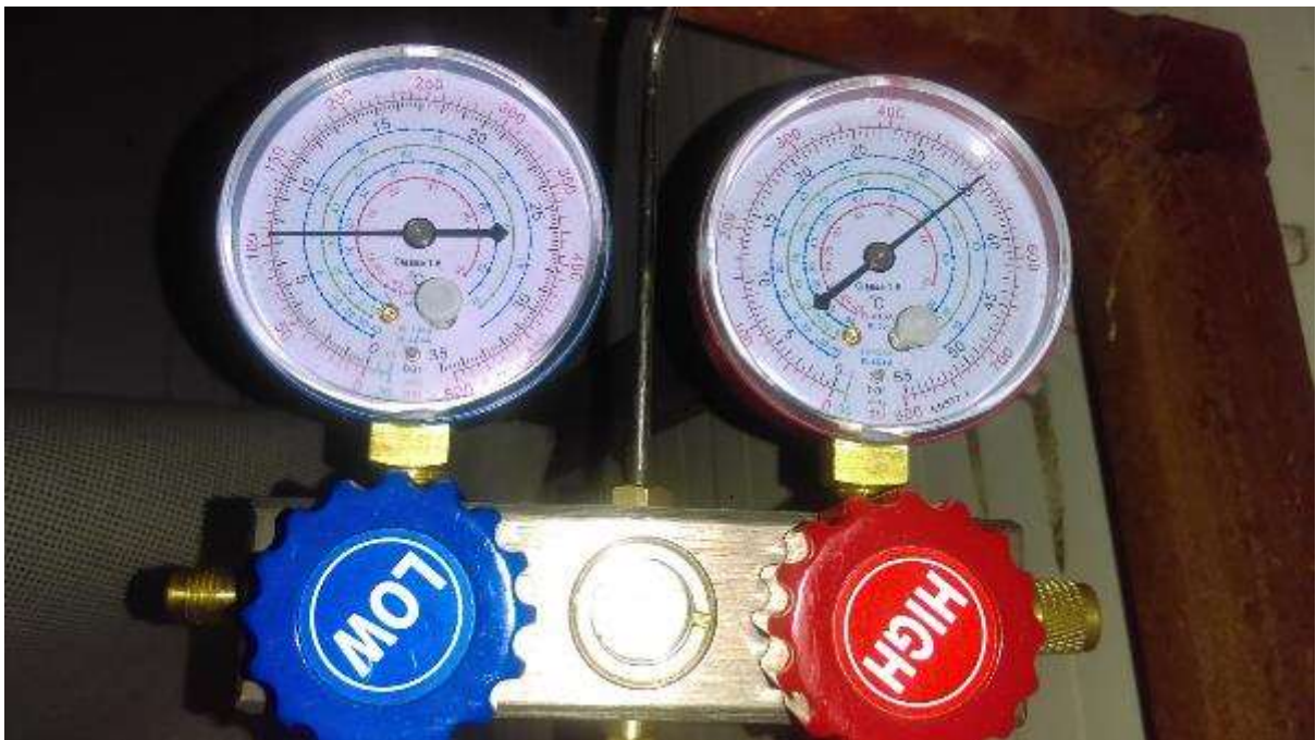
Figure 58 Experimental study bench cold and hot gas lines pressure measurement example
