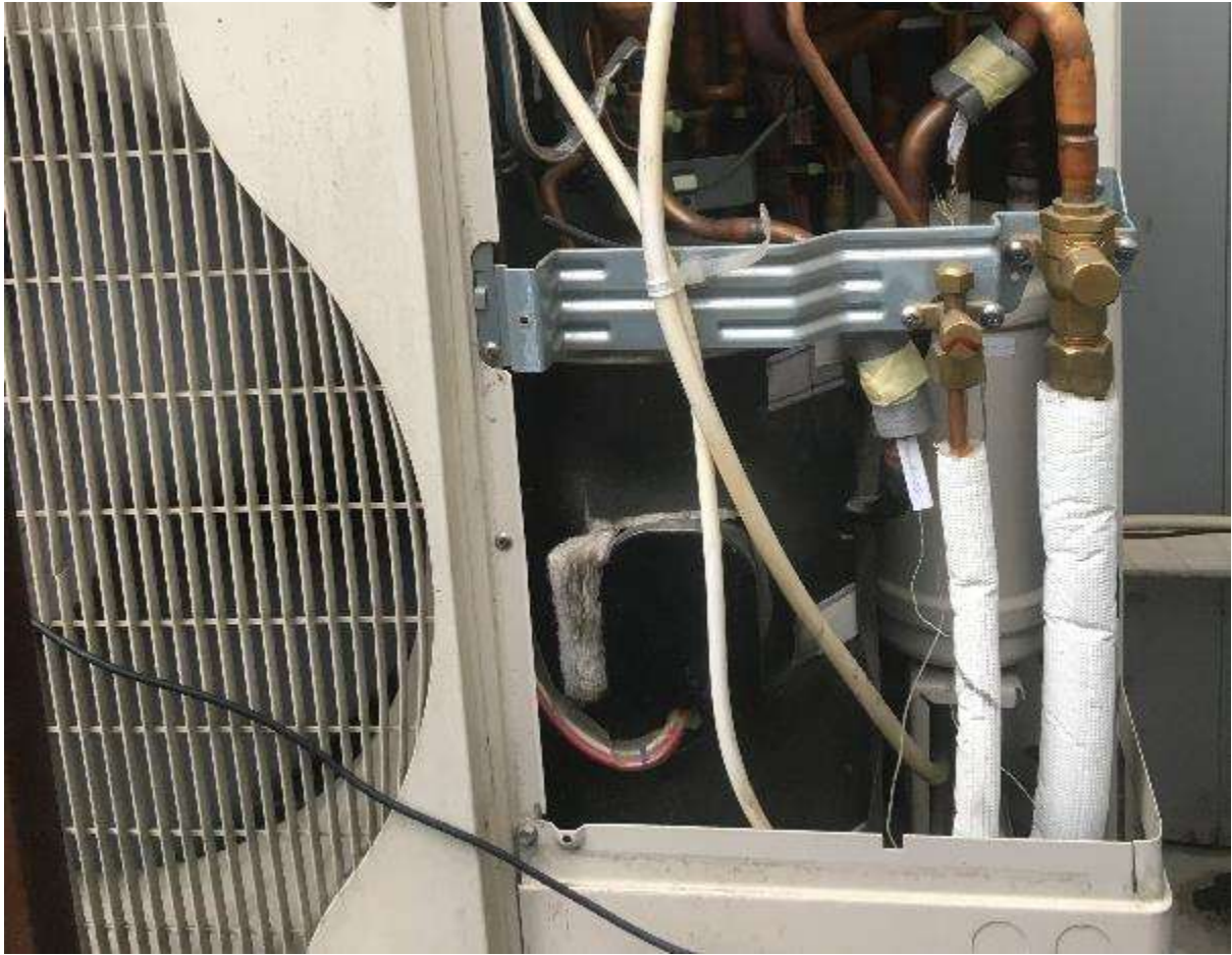
Figure 47 Experimental study bench refrigerant liquid and vapor connection lines
