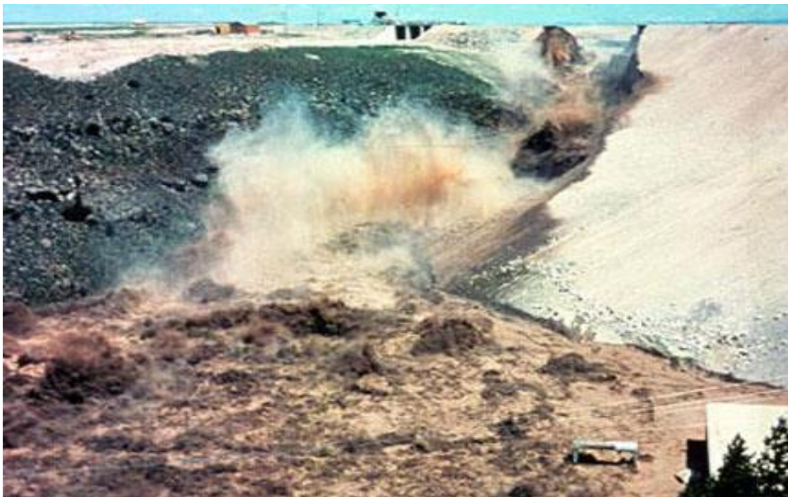
Figure 7. Photograph of Teton Dam: leak has enlarged and widened, crest (bridge) has collapsed, the outflow exceeds 28,300 m 3 /s eroded all the dam fill entirely, [7].
