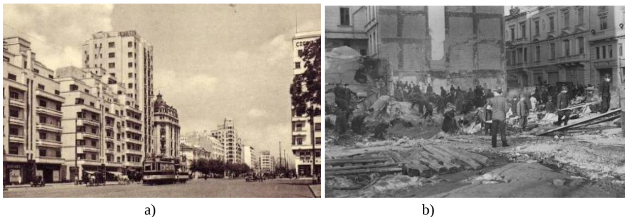
Figure 8 – Carlton Block: a) before the 1940 earthquake; b) before the 1940 earthquake
