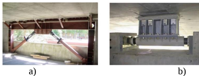
Figure 5.18 - a) Pall-type seismic motion damping device, used in the composition of "X" braces - Patient Tower, Seattle, USA; b), c) Damptech seismic motion damping device, used in the composition of bracing - Yaguriji Temple, Japan [99]
