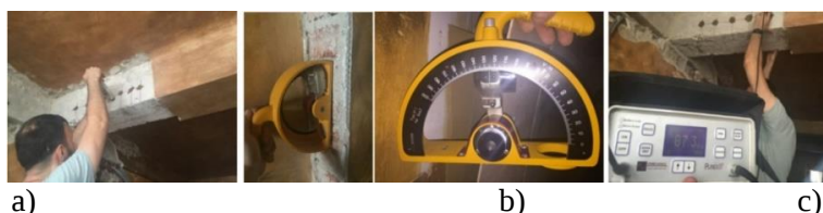
Figure 6.11 - a) Sclerometry method used to determine the compressive strength of reinforced concrete; b) sclerometry method (8x14x28 cm brick masonry elements); c) Ultrasonic method for determining the quality / possible defects of reinforced concrete [119]
