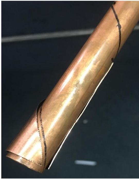
Figure 4-11. Locate the copper pieces on the pipe.
