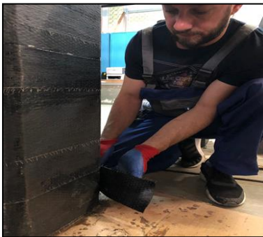
a) Wrapping CFRP strips.
