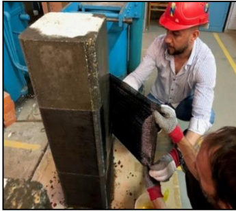
c) Applying epoxy resin MapeWrap 31
