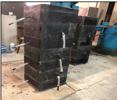
d) Insert MapeWrap FIOCCO cord in each hole.
