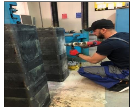
c) Drilling holes for the anchors.
