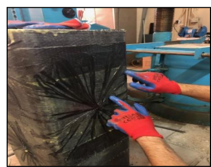
f) Apply a coat of MapeWrap 31 on the substrate then splay all the fibers
