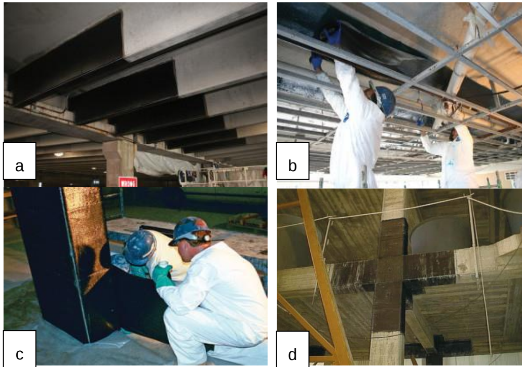
Fig. 5: Typical applications as strengthening materials of RC structures. (Source: Teach Engineering Lessons).
