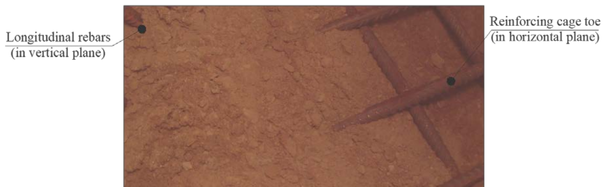
Figure 23. Pile base after installing the pile reinforcing cage
