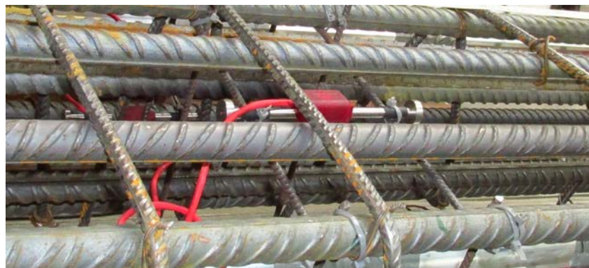
Figure 8. Embedded strain gauges constructive sketch [9] and example of installation on the reinforcing cage of a prefabricated pile (construction site on The Netherlands)
