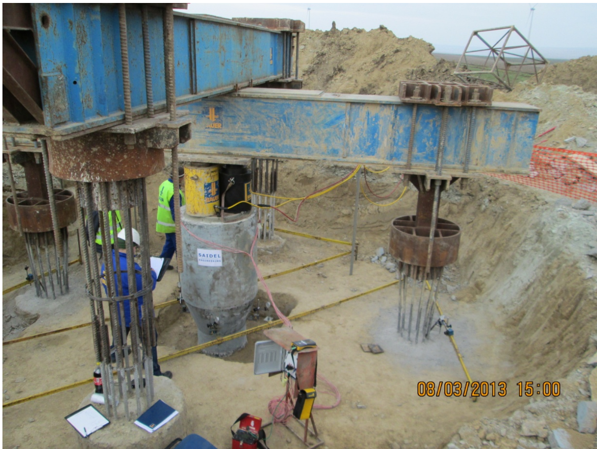
Figure 16. Axial compression load test overview PP2
