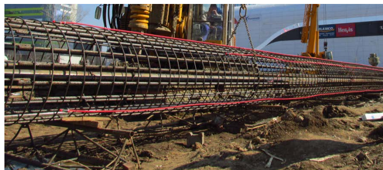
Figure 3. Reinforcing cage ready for installation
