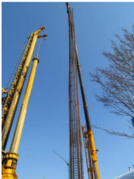
Figure 2. Reinforcing cage
