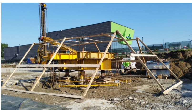
Figure 24. Axial compression load test overview PP3
