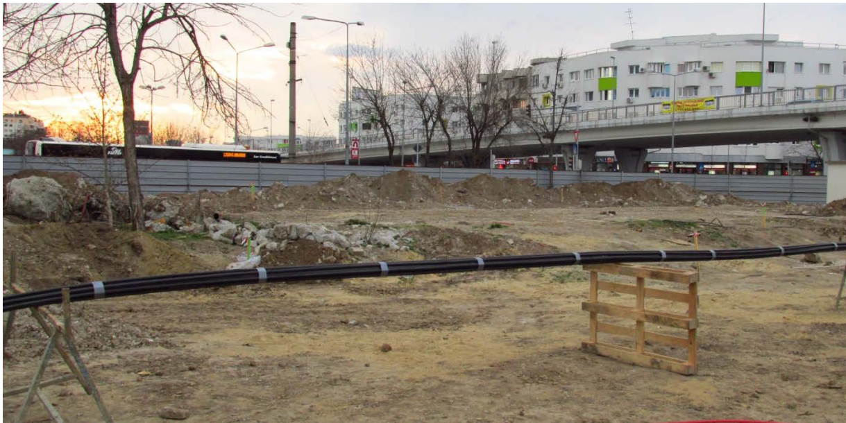
Figure 9. Rod extensometer ready for installation in pile PP1
