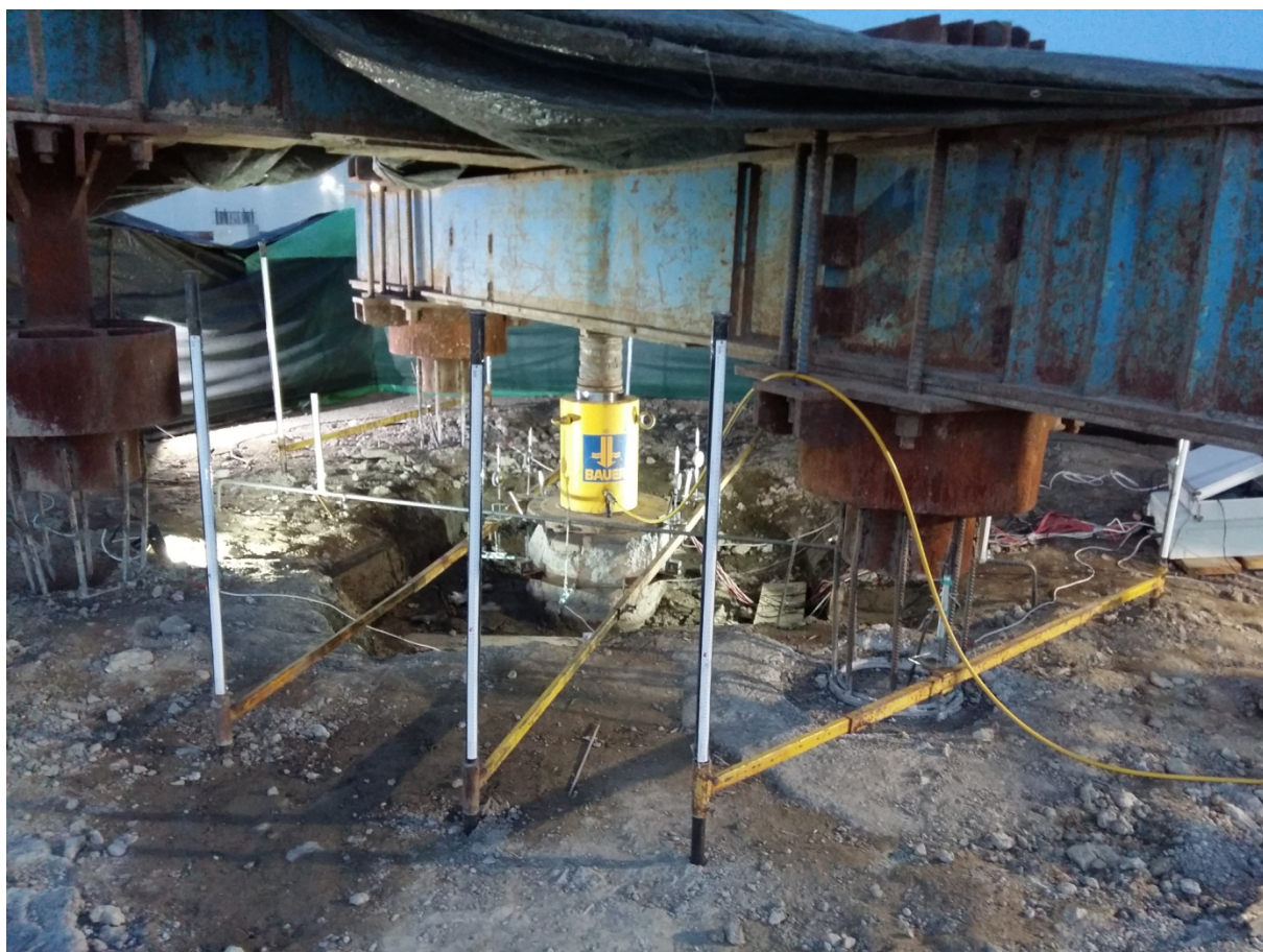
Figure 34. Axial compression load test overview PP4
