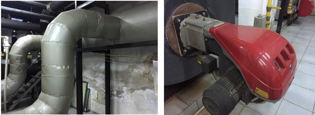
Fig.27 Noise protection solutions in boiler plant
