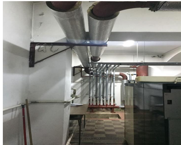
Fig.38 Noise protection solutions in boiler plant
