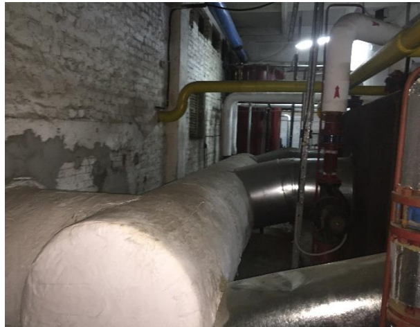
Fig. 9 Noise protection solutions in boiler plant
