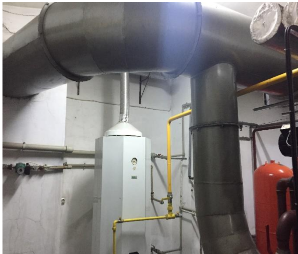
Fig.38 Noise protection solutions in boiler plant
