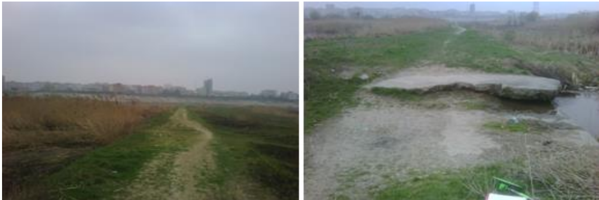
Figure 17. Photos from the field with the top of abandoned collector
