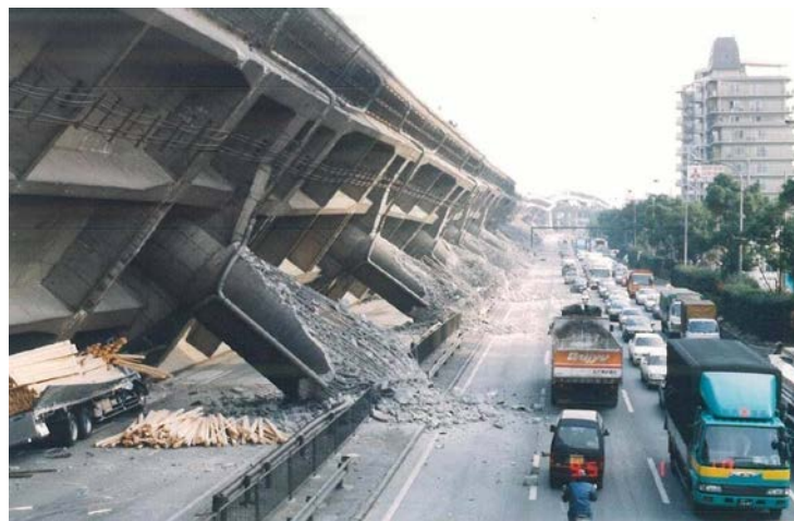
Fig. 1 Collapse of bridge nr. 3 on the Hanshin Motorway (Kobe 1995)
