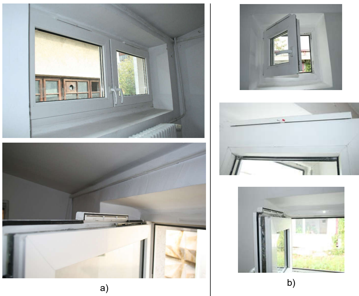
Fig. 3. The window kitchen a) and the bathroom window b)
