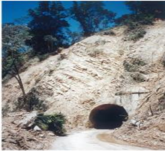
Fig.4.8. The portal of the Haguro tunnel
