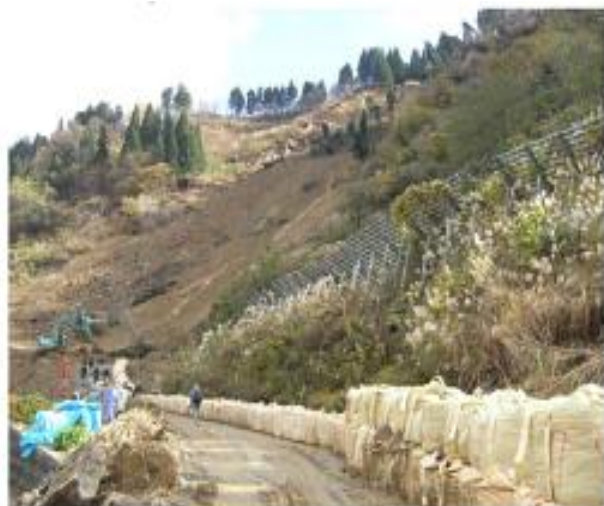
Fig.4.11. Land sliding near the western entrance of the Haguro tunnel.
