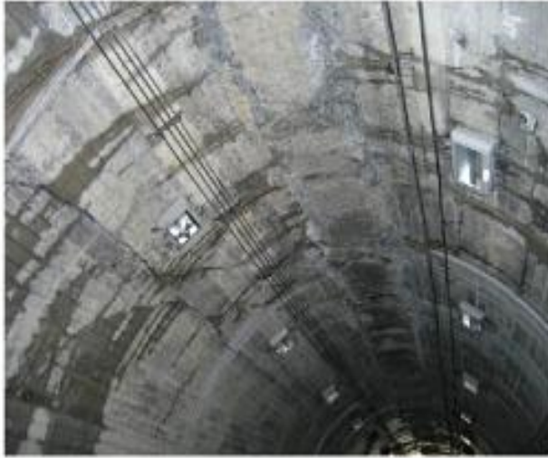
Fig.4.10. Extended longitudinal cracks in the Haguro tunnel.
