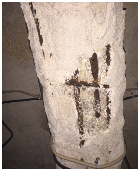
fig .4.1.2.degradari structura cladire S+P+3E -1930 subsol - fara ventilatie-beton complet exfoliat
