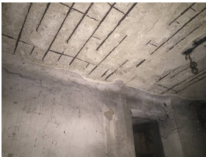
fig .4.1.2.degradari structura cladire S+P+3E -1930 subsol - fara ventilatie-beton complet exfoliat
