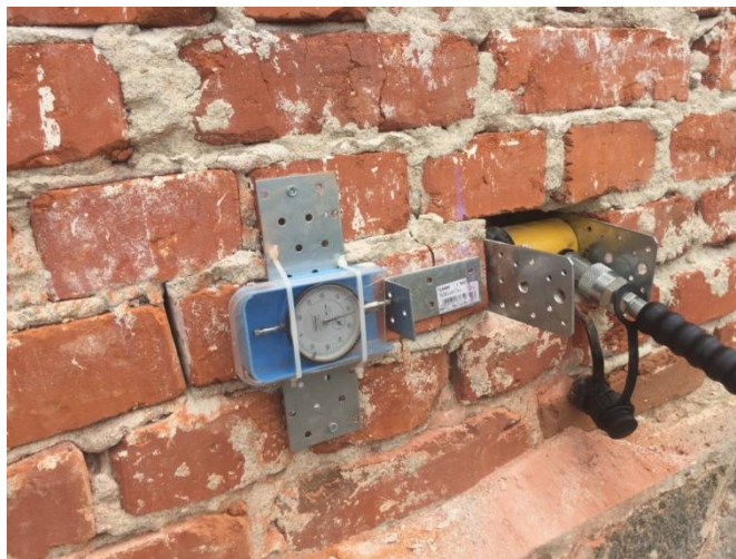
FIG 6 .SHOVE TEST -SHEAR MORTAR VALUE STUDY -
