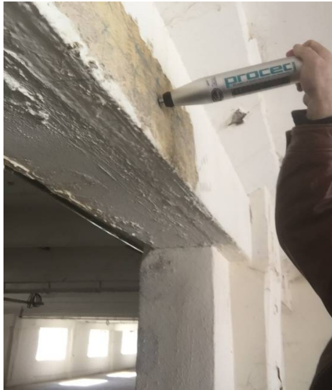
FIG.3 SCHMIDT HAMMER TESTING ON BEAM -MEDIUM TIPE CONCRETE
